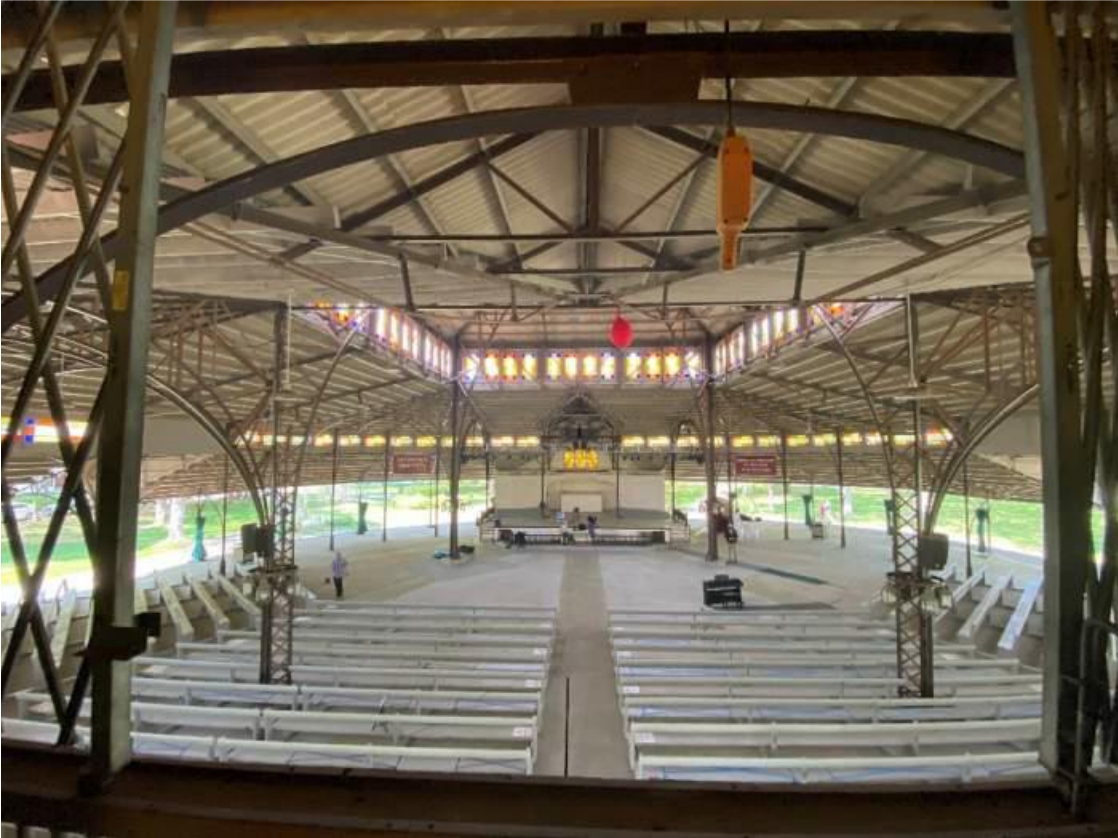
1. General Interior View
