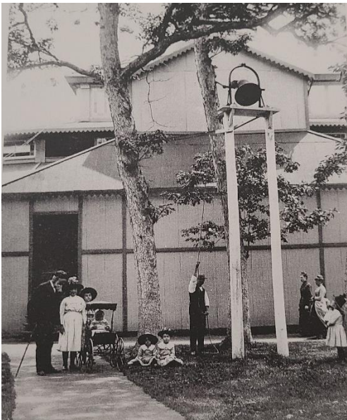
3. Historical Accessory Structure from pre-1901 in the Exterior Stage Wall location
