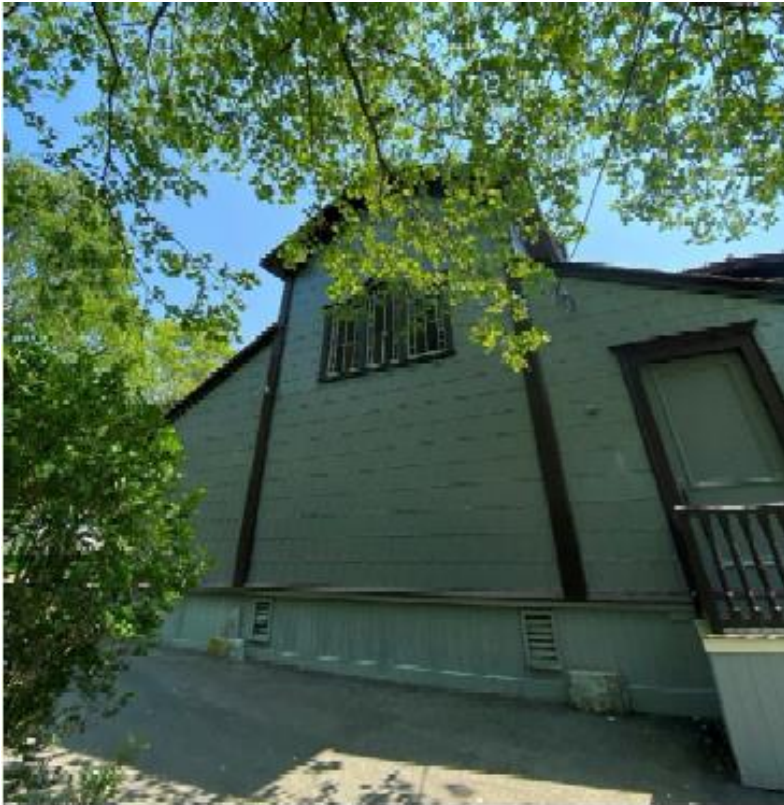
2. Exterior Stage Wall to which addition will be affixed
